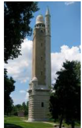
Compton Water Tower
